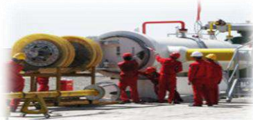
Pig Launcher and Receiver
