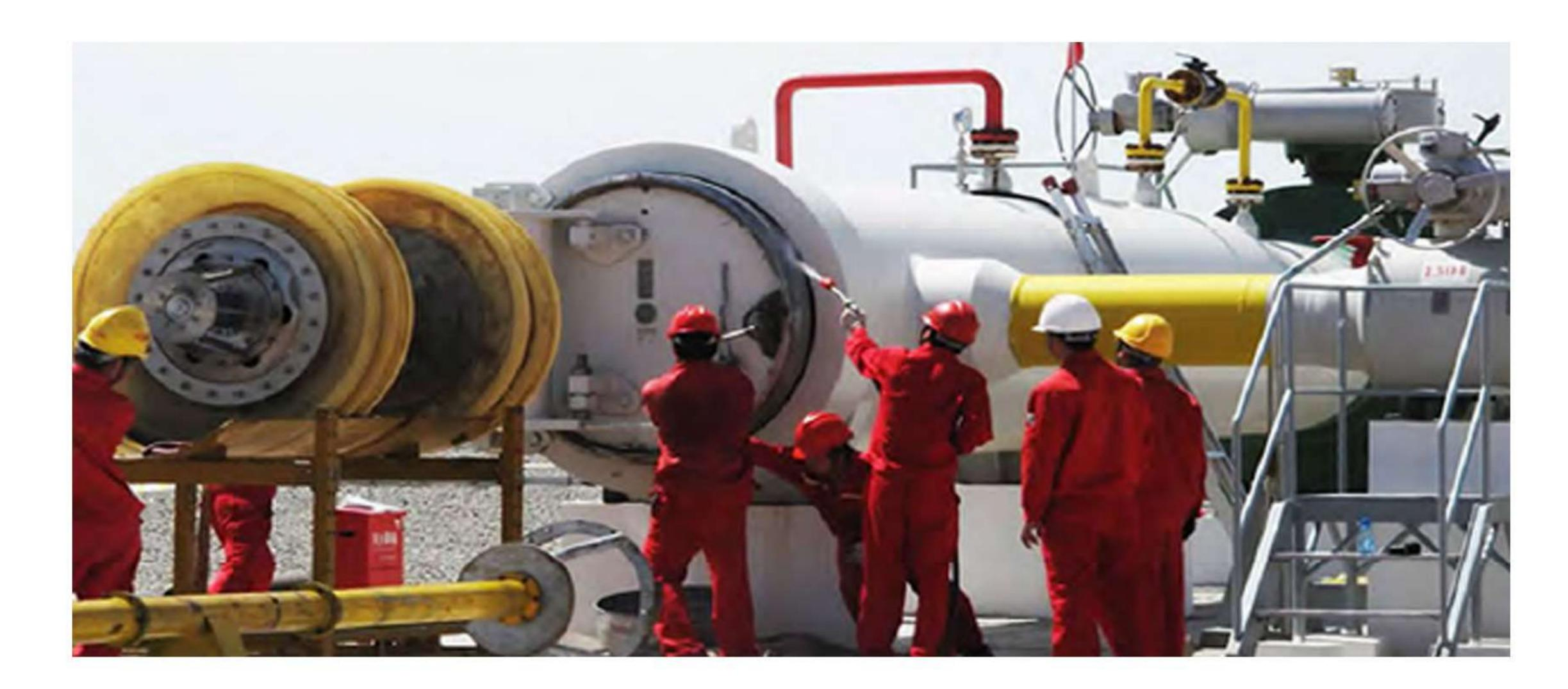
Pig launcher & receiver are important parts of pigging equipment on long distance pipeline, which is installed on both ends of pipeline to launch or receive the pig. It mainly consists of quick opening closure, barrel, reducer, and saddle support. Pig launcher & receiver shall assemble vent valve, safety valve and pressure gauge and other parts.
