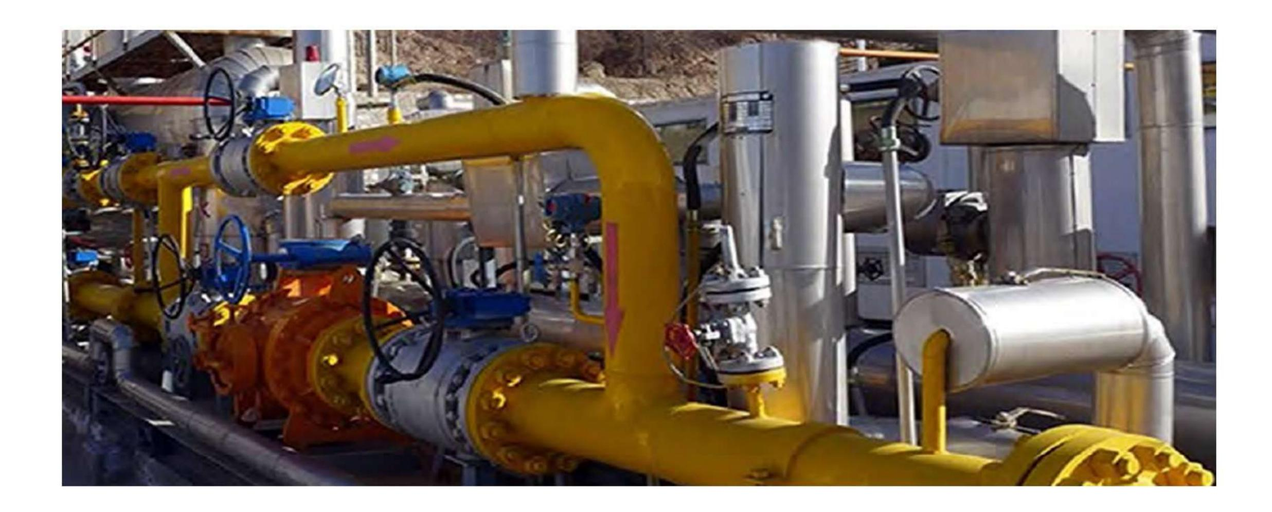
A set of gas production and gas well to summarize system, gas-water separation system, drainage and blowdown Flash tank system, piping pigging system, output metering systems, use gas decompression system equal to one and integrating new digital automatic control of skid-mounted.
