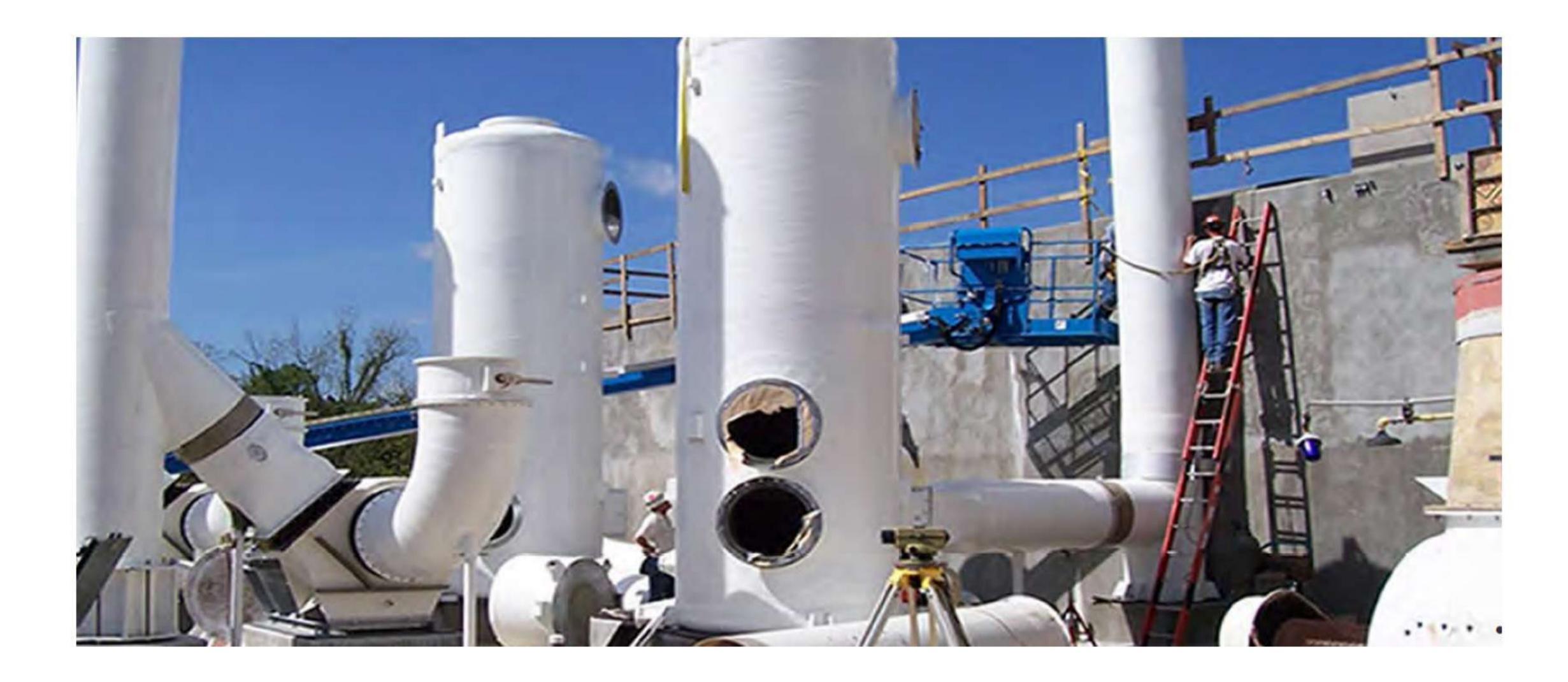
Gas Scrubber removes traces of liquid droplets from gas streams to protect downstream equipment from damage and failure.
