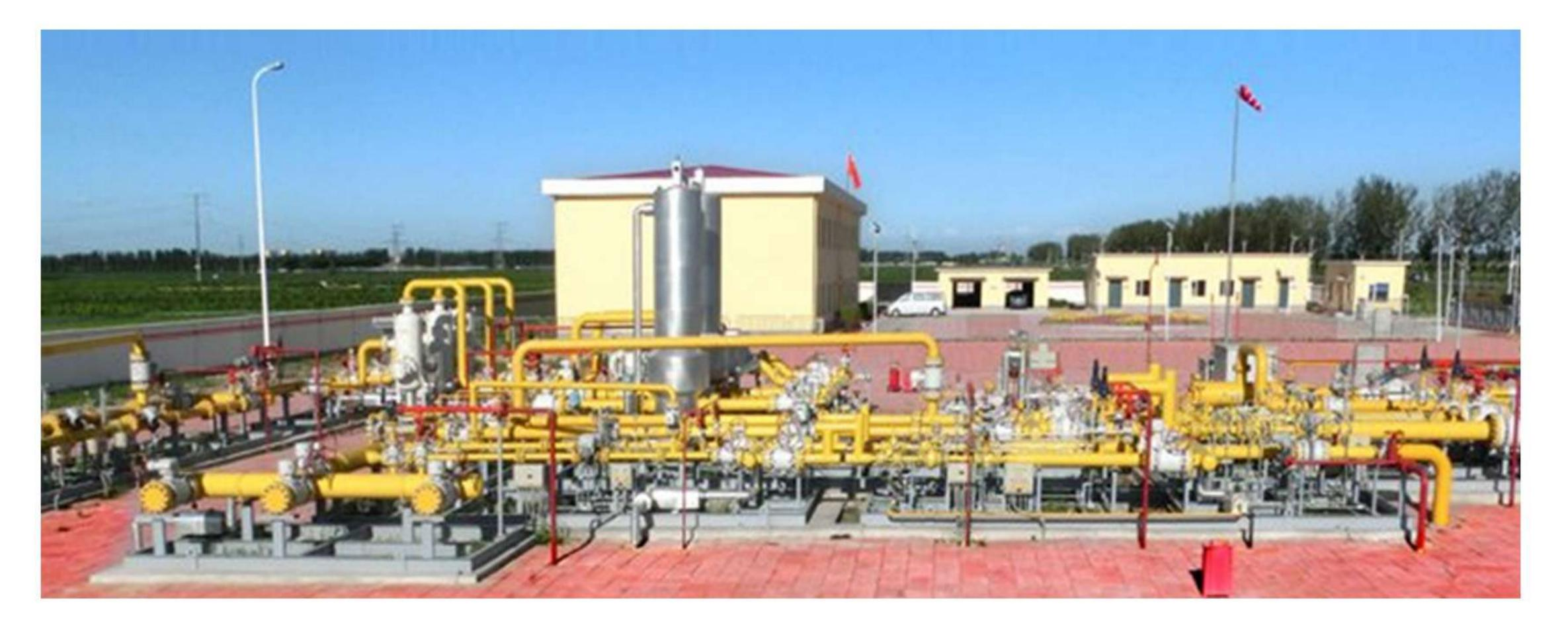
City gas station/ storage and distribution station is a large skid-mounted regulator station specially designed for city gas. It is a gas supply equipment to civil and industrial users after gas filtering, regulating. metering peak shaving and odorizing.
