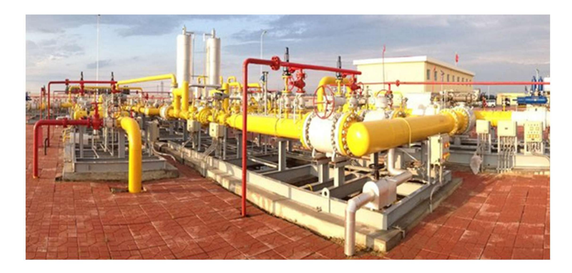
The skid-mounted pressure reduction metering station industrial gas) is a regulator station specially designed for industrial users, including gas power plant (gas turbine, gas boiler and other gas supply facilities), fertilizer plant, ceramic plant, carbon plant, glass factory and other enterprises. It is a gas supply equipment to industrial users after gas filtering, regulating and metering.
